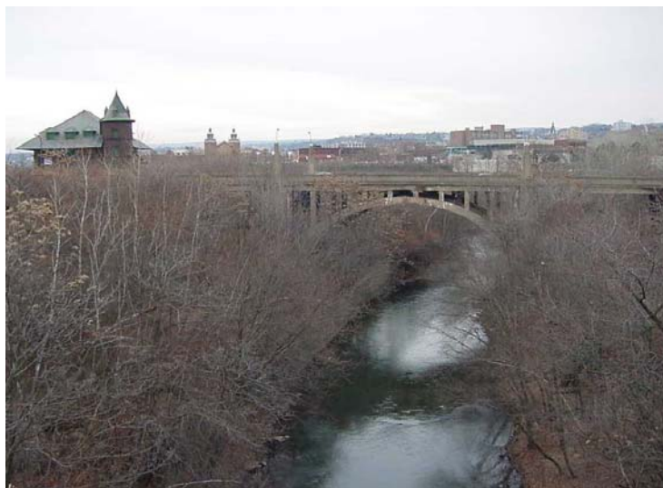
Lackawanna Ave. bridge with former CNJ Passenger station at top left
